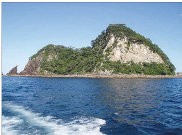
Figure 11. Recent rockslides were evident through the fringe forest on the talus slope at the foot of the summit cliffs by the western end of Motueka. Photo looking SE: 1 Mar 2005.
